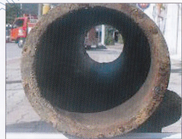
5 years after the installation (October 4, 2007)
