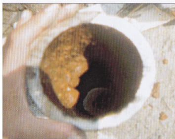
before the installation (October 17, 2002)
